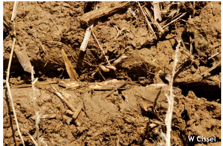
"Slug highway" left when the seed trench isn't closed all the way.
