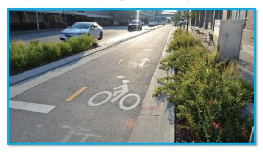
**IMAGE 25:** Example of bioswales integrated with bicycle lanes. <sup>122</sup>
