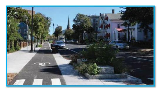
IMAGE 17: Example of raised bike lane beside pedestrians and separate from motorized vehicles. 112
