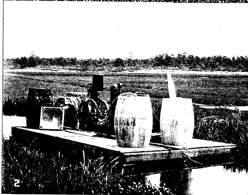
PLATE VII.— PIPING (1) AND SPRAYING OUTFIT ON FLOAT (2) FOR SPRAYING A LARGE BOG FROM ONE CANAL. (Used primarily for cranberry diseases.)
