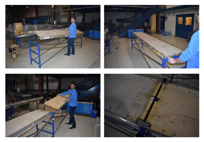
Figure A3. Pictures showing installation of the scaffold planks.
