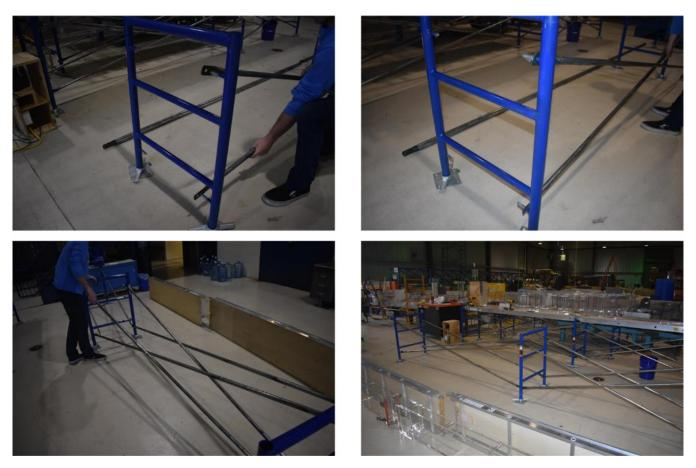
Figure A2. Pictures showing cross brace installation.
