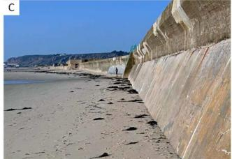
*Figure 24. Examples of methods to protect beach using hard structures. A) Offshore breakwater, B) Gabion structures, C) Seawall.*
