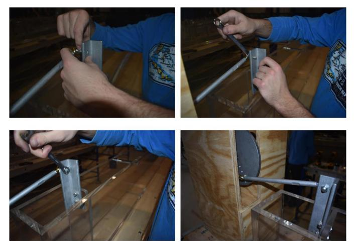
*Figure A13. Pictures showing attachment of linkage arm to wave flume paddle arm.*
