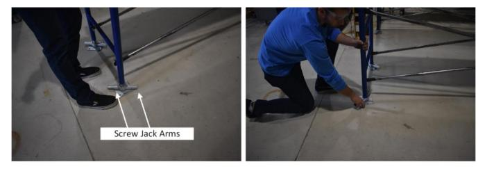
Figure A4. Pictures showing jack screw adjustment.
