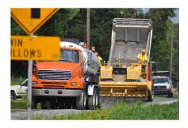
the application type, a chip seal can extend the life of the pavement by 5-7 years or more and traffic can usually be restored within an hour or two of application.
