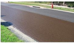
The final surface of slurry seal needn't be particularly pretty to be functionally effective, as long as good coverage is achieved and no ridges are left that can trap water at the surface. However, a thoughtful application that results in a smooth surface will be more appealing to residents of the neighborhood and will go a long way towards them accepting the product aesthetically. Translation: greater acceptance = less complaints = less meetings = being left alone to do your job.
