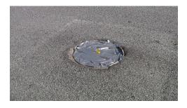
emulsion "breaks" (in reference to the weak water/oil bonds breaking down), the water usually evaporates, and the surface turns jet black. In August, this can happen very quickly, but in October under cloudy skies, this can drag on. Indeed, the released water may not evaporate; it may sit at the surface if it cannot run off naturally. Warm, breezy days with low humidity are ideal. Rain or wet surface conditions are a non-starter.
