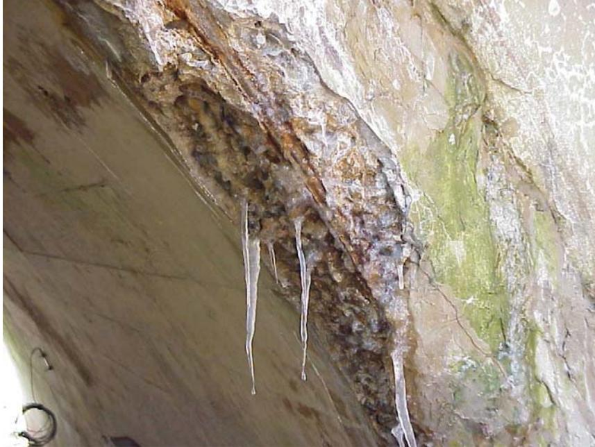
**Photograph 3. Spalling of Concrete Along the Edge of the Bridge.**
