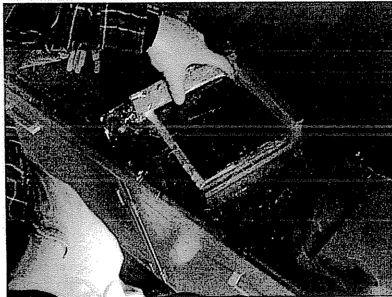
Figure 3.10 Placing release film over completed panel to prevent bonding to additional panel or forcing plate.
