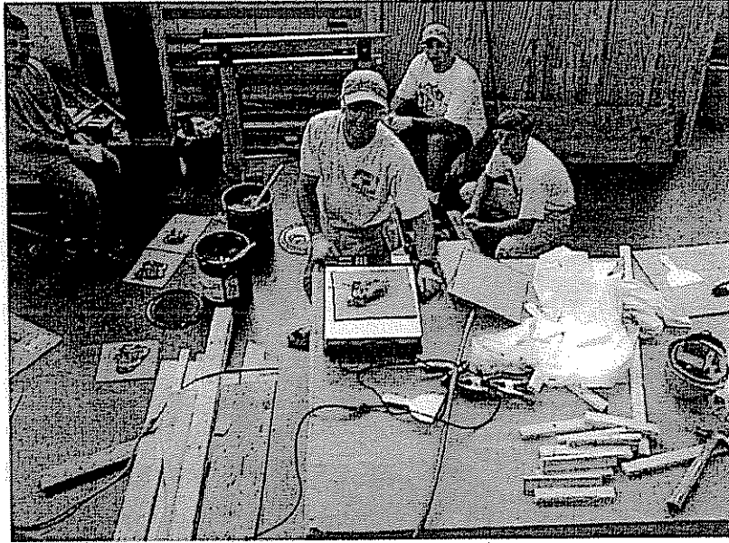
Figure 5.9 Weighing the parts of adhesive to ensure a proper mix. On the floor in the background, note the individual components awaiting mixing.
