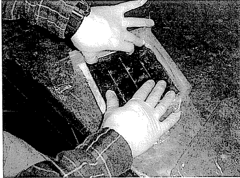
Figure 3.11 Securing composite strips and ensuring that none have slipped or rotated out of desired alignment.
