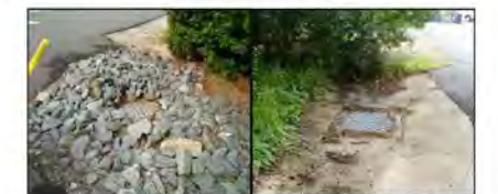
Figure 9. Inlets surrounded by rip-rap and concrete in N4 (South Bethany) that can be modified to remove the impervious cover and include grass/native vegetation pretreatment.
