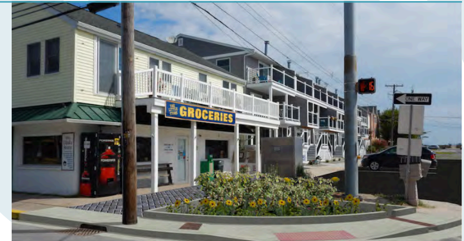
Bio-retention Reservoir Photo: Delaware Center for the Inland Bays
